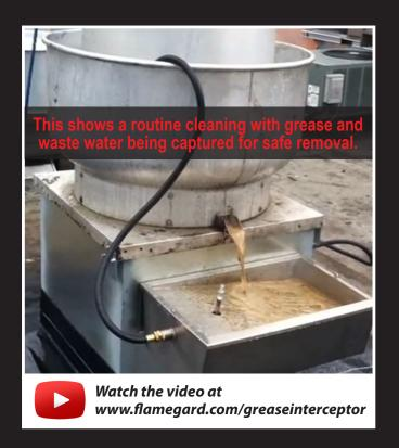
Prevents grease and harmful chemicals from entering the sanitary or ground water system.
